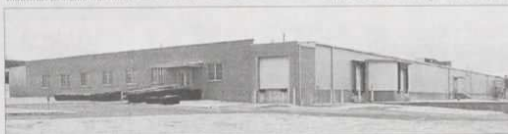
Gamco USA has leased this 66,000 square foot building on South Sam Houston Blvd. in Houston. The firm has an option to purchase it from the Houston Industrial Development Authority. The federal government has given its blessing to the proceeds to be used for construction of another industry building in Houston, according to the City of Houston.
